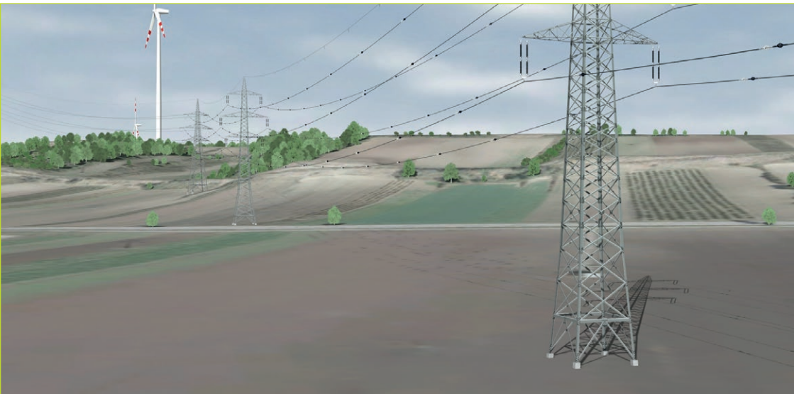
High voltage power line network and wind power plants in the east of Austria.
